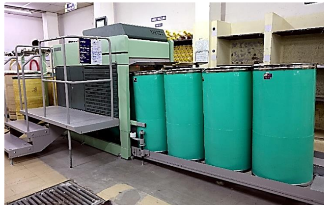
A view of new “Rieter – RSB D50” Draw Frame Machine installed in our Unit-I at Rajapalayam.
